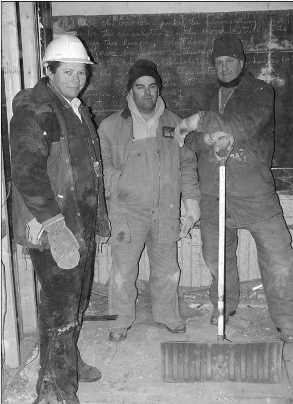
Tymen Van Stryland, Jeff Bray and Dave Johnston were three of the Vilida Construction workers who uncovered a century-old pine wood chalkboard this week under the drywall of an old schoolhouse on March Road.
